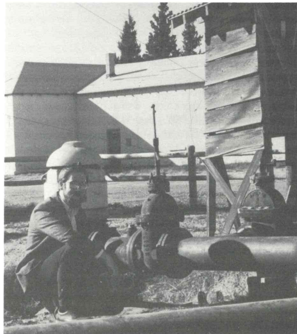
Calvin Lashway inspects NMSU Well No. 7, which was originally drilled in 1935. The Seed House (background) has served the Agricultural Experiment Station since at least 1895. Several early wells were drilled in the vicinity of the Seed House, which today is used as a dry lab and for storage.
